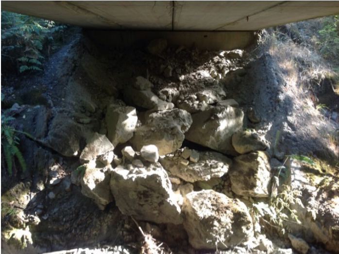
Left Bank Abutment when facing downstream
