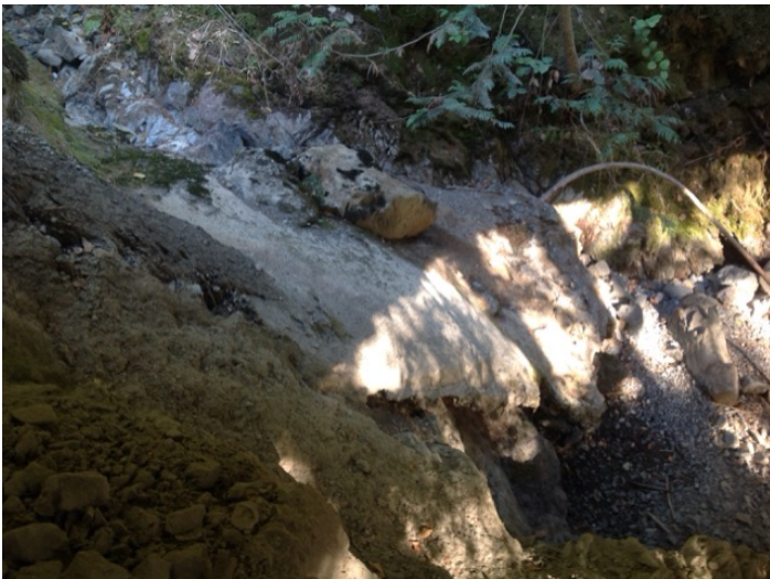
concrete on right bank
