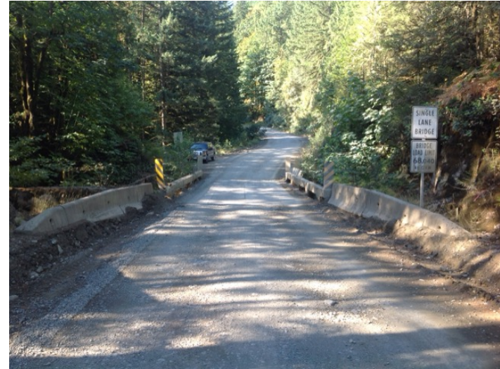
Approach from Left Bank when facing downstream
