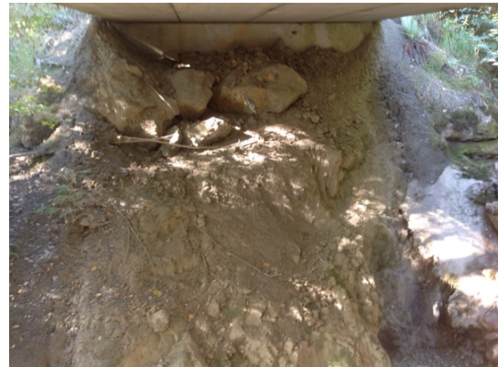
Right Bank Abutment when facing downstream
